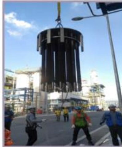
Removal from the Pressure Vessel
